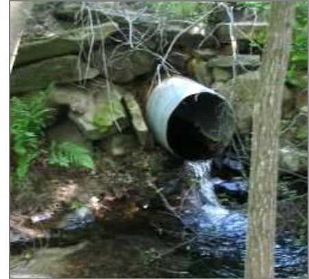
A “perched” culvert on River Road in Windsor, preventing fish passage and resulting in scour at the outlet. (CEI photo)
